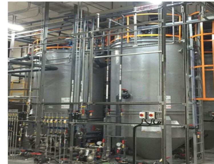
As Batch Reactor
